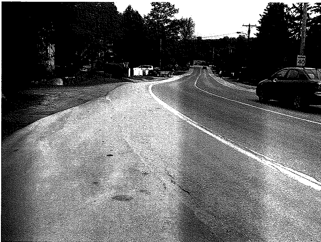
Sta. 42 + 825 approximately looking north.
