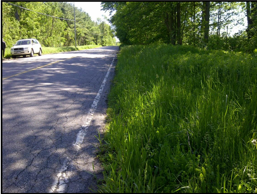
Figure 9 Olde Base Line - Very Narrow (or No) Shoulder, Tall Grass, Extensive Pavement Edge Cracking
