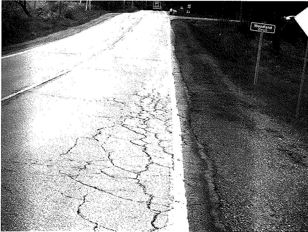
Sta. 41 + 500 approximately looking north.
