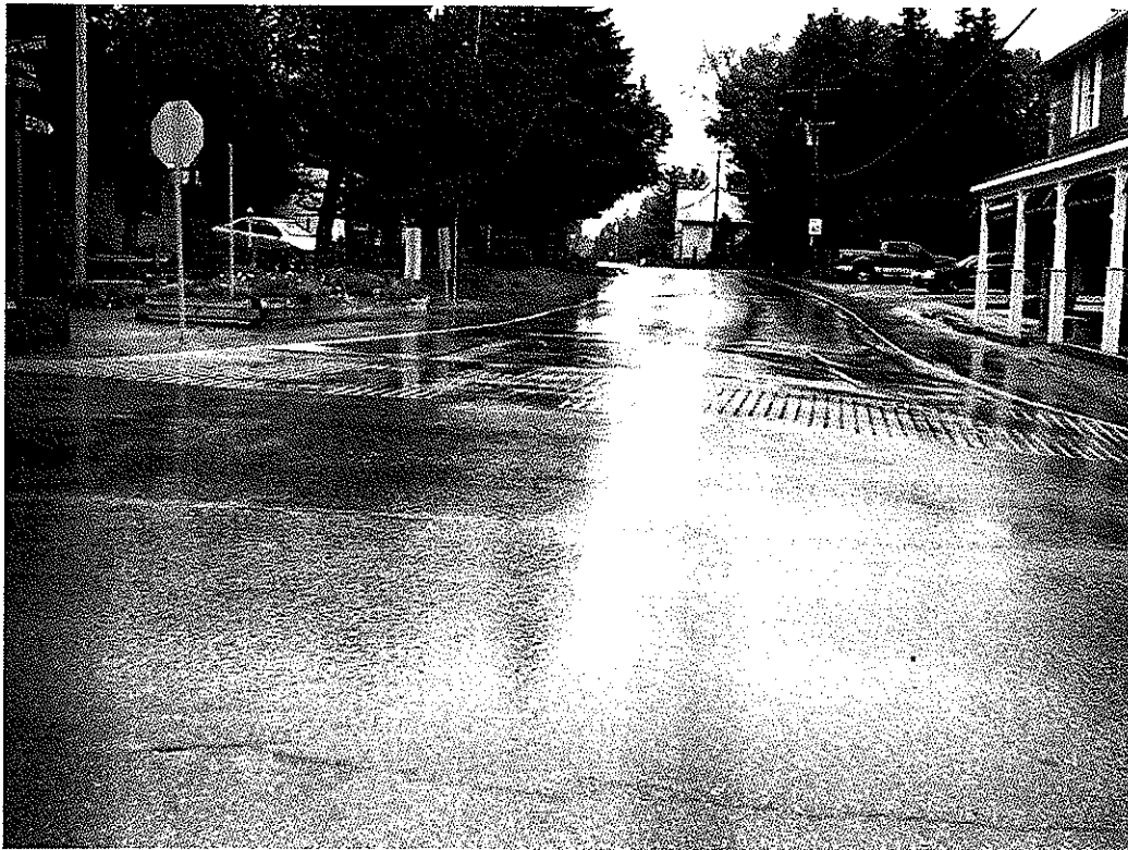
Sta. 2 + 050 approximately looking west.
