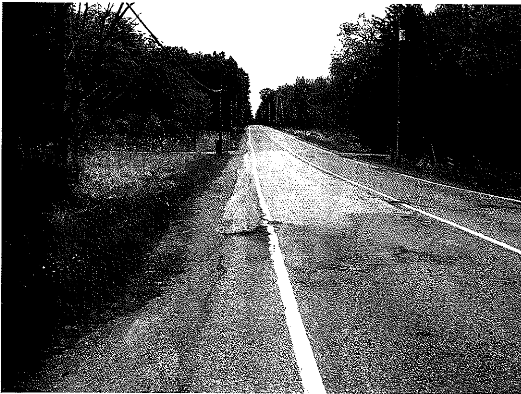
Sta. 38 + 000 approximately looking south.
