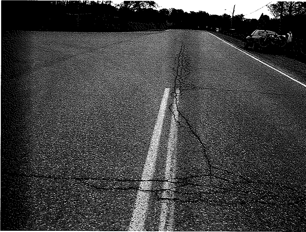
Sta. 0 + 000 approximately looking east.
