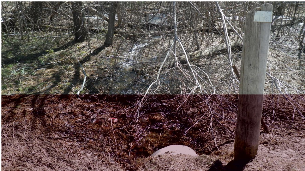
Photo 18: View looking upstream of culvert inlet.
