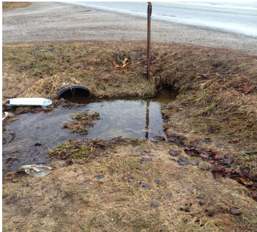
Photo 9: View looking upstream at culvert outlets.
