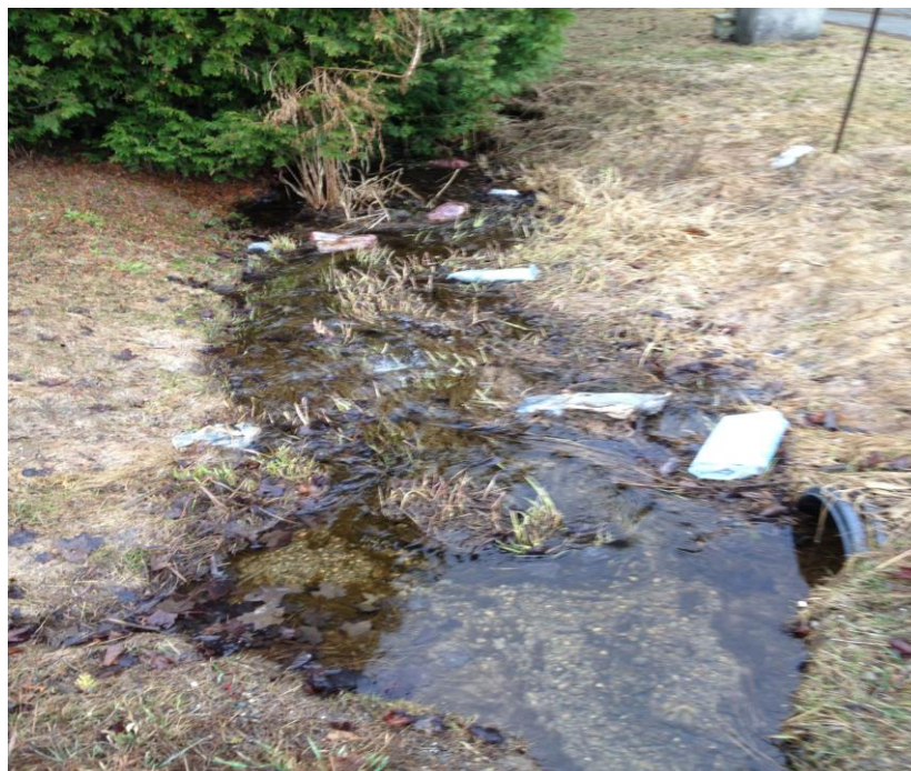
Photo 10: View looking downstream of culvert.
