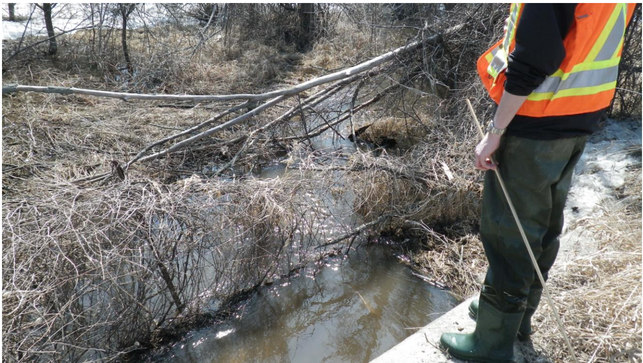
Photo 20: View looking downstream from culvert outlet.
