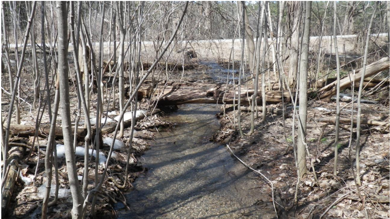
Photo 17: View looking upstream towards culvert outlet.
