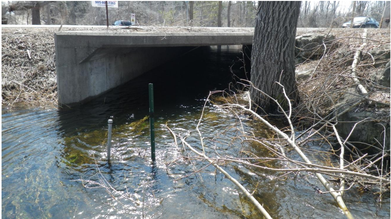
Photo 21: View looking downstream towards culvert inlet. Level logger is present just upstream of culvert.
