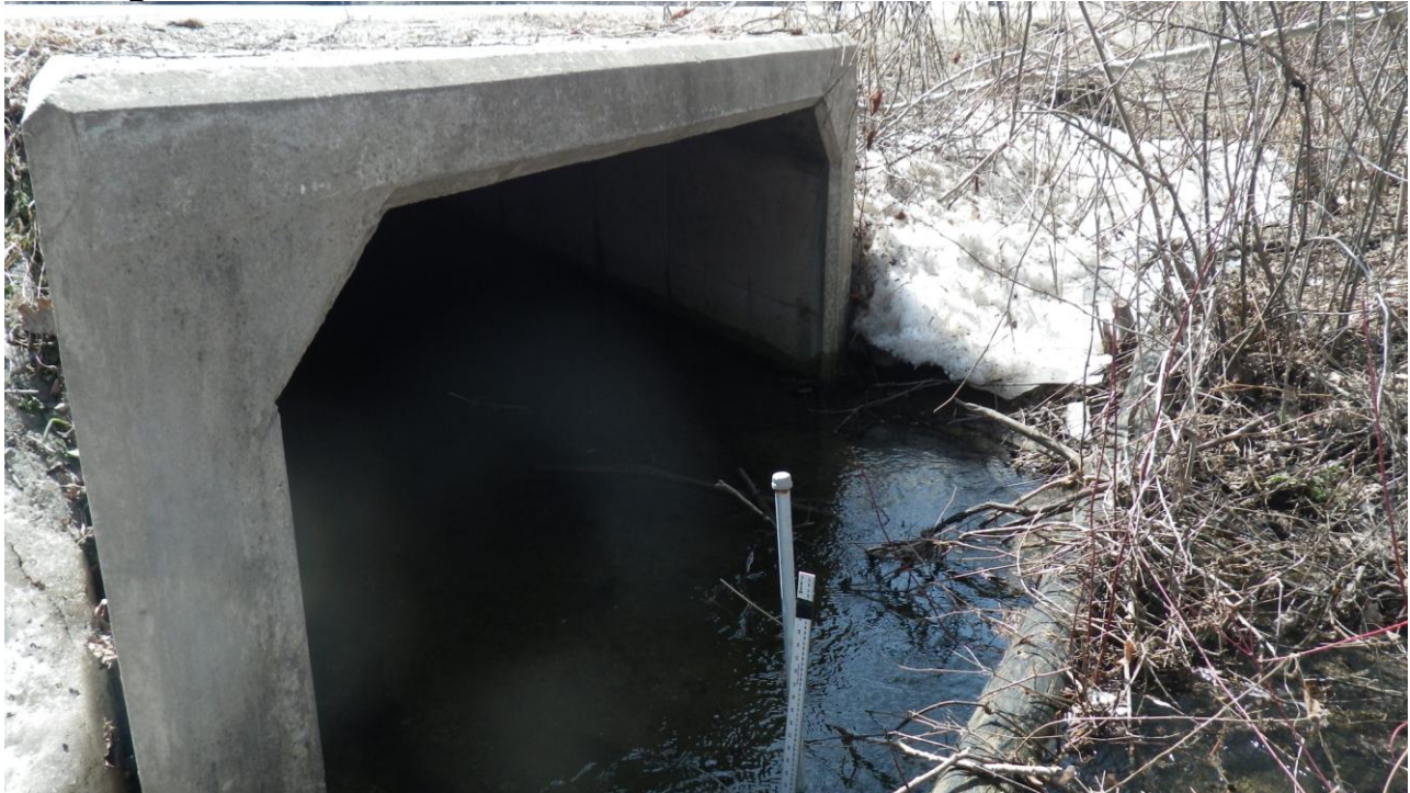
Photo 19: View looking downstream at culvert inlet. Level logger is present just upstream of culvert.
