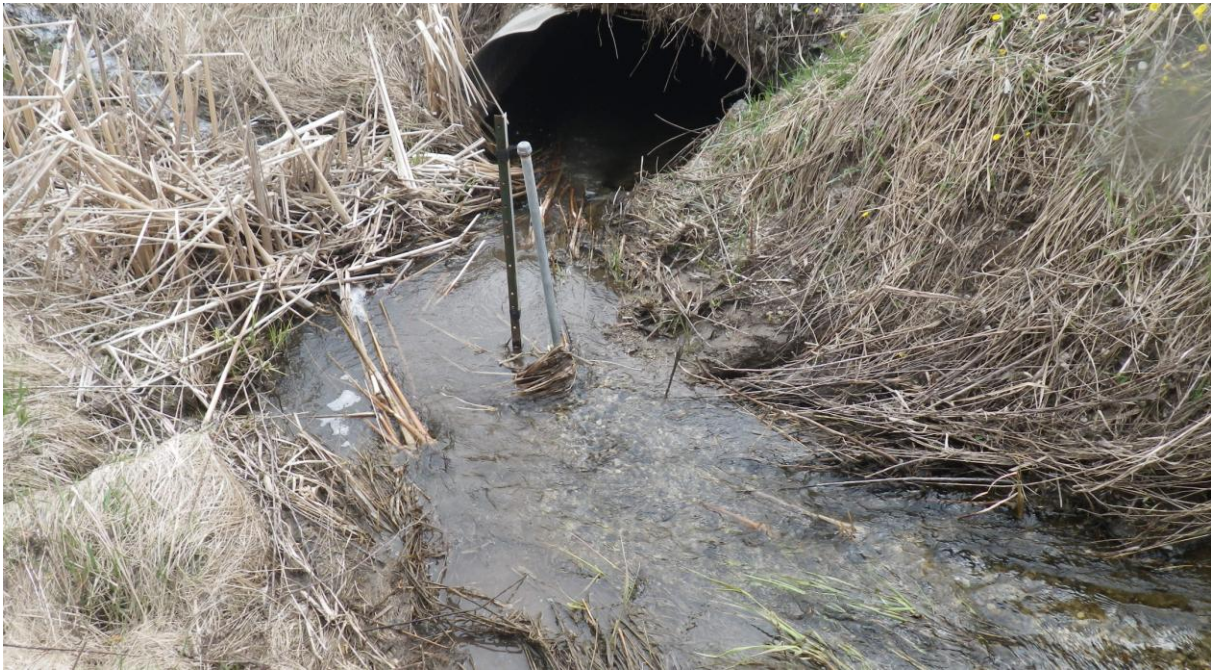
Photo 11: View looking downstream towards culvert inlet. Level logger is present just upstream of culvert.
