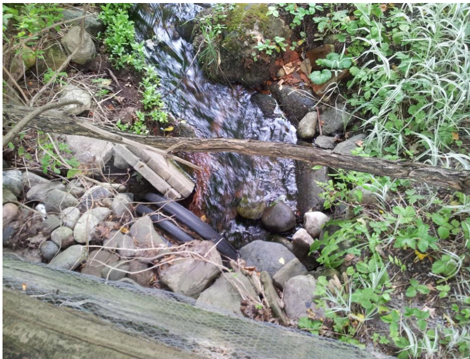
Photo 6: View looking just downstream of the online pond at culvert inlet.
