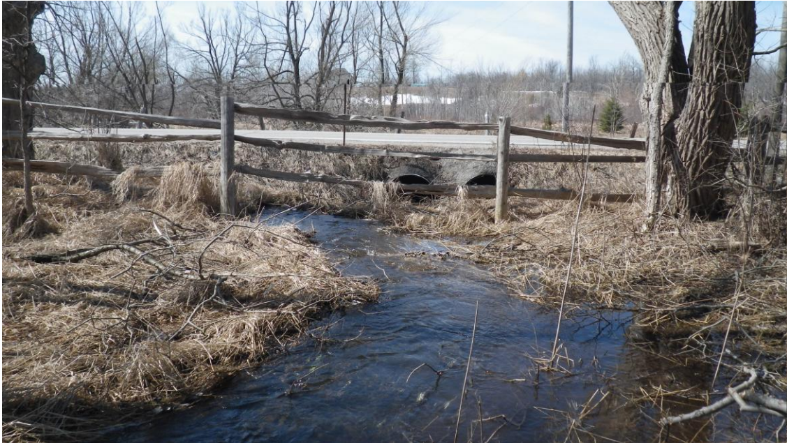
Photo 1: View looking downstream towards twin corrugated steel pipe culvert inlets.
