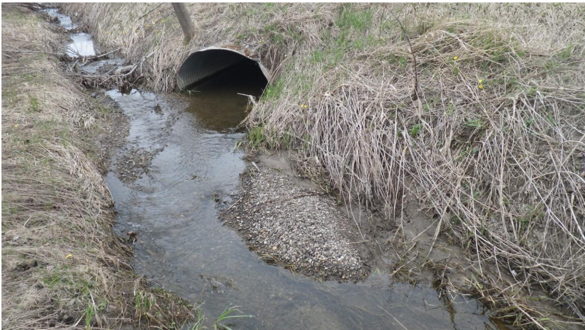
Photo 12: View looking upstream towards culvert outlet.
