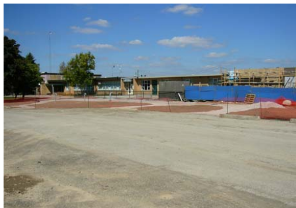
Belfountain School Construction.
